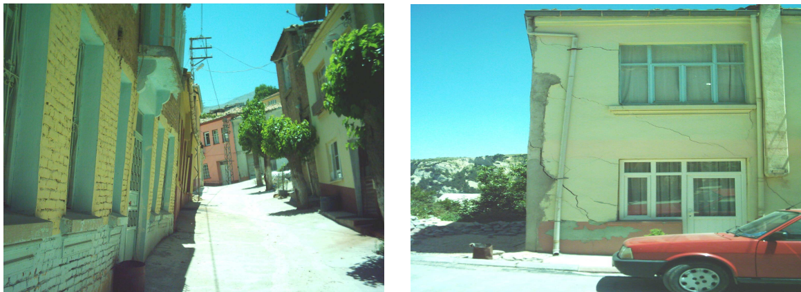
Photo 3.a. and 3.b. vertical inclination and fissure on some houses
